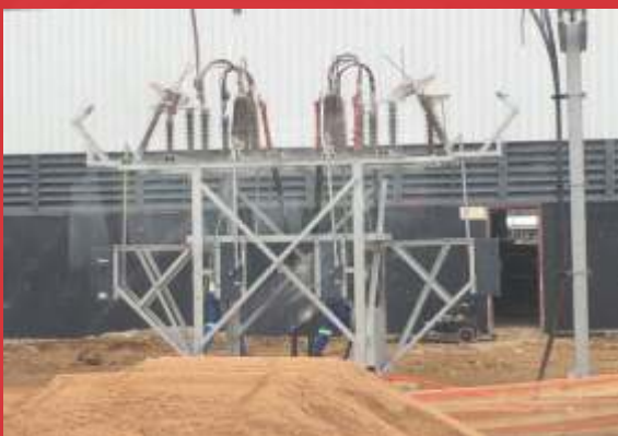
Change-over Yard Switch on-site at Gibela
